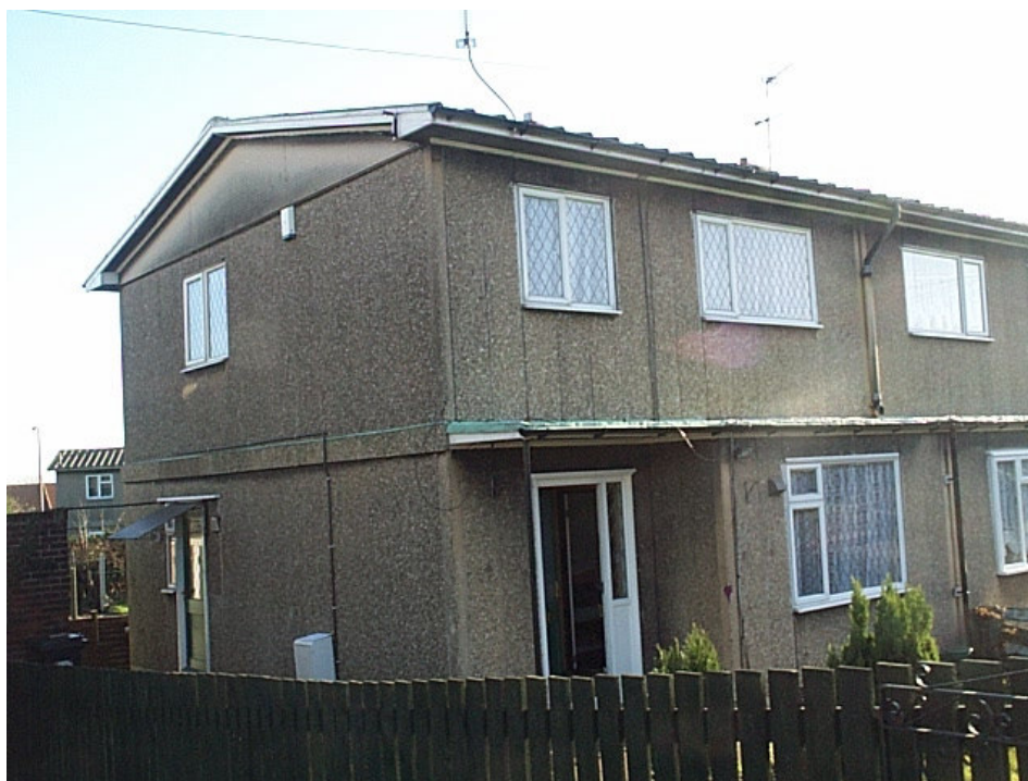
Photograph 1 – Typical Front Elevation of Tarran Newland House
